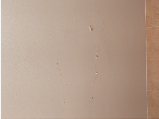
Hazard: Bathroom 2 | Ceiling | Deteriorated Paint Hazard: Bathroom 2 | Wall | Deteriorated Paint
