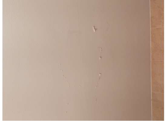
Hazard: Bathroom 2 | Ceiling | Deteriorated Paint Hazard: Bathroom 2 | Wall | Deteriorated Paint
