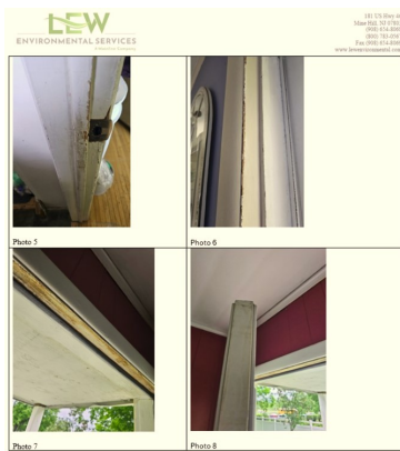
Hazard: Living Room | Door | Deteriorated Paint
