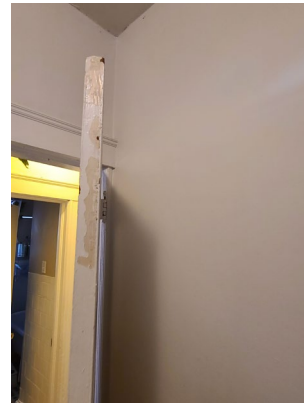
Hazard: Bedroom 2 | Door Jamb and Casing | Deteriorated Paint
