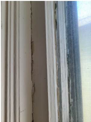
Hazard: Bedroom 1 | Door, Jamb and Casing | Deteriorated Paint
