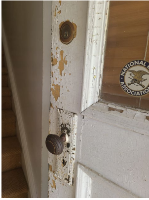
Hazard: Stairwell 1 | Door and Door Frame | Deteriorated Paint
