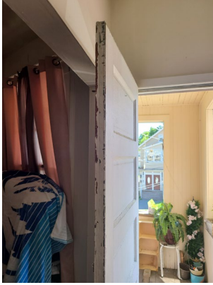
Hazard: Bedroom 1 | Door, Jamb and Casing | Deteriorated Paint
