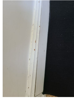
Hazard: Stairwell 1 | Baseboard | Deteriorated Paint
