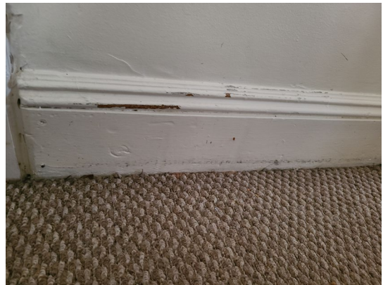
Hazard: Stairwell 1 | Baseboard | Deteriorated Paint
