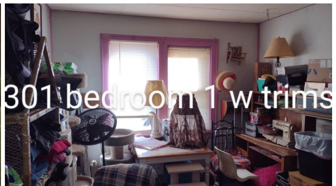
Hazard: Bedroom 1 | Window trims | Deteriorated Paint
