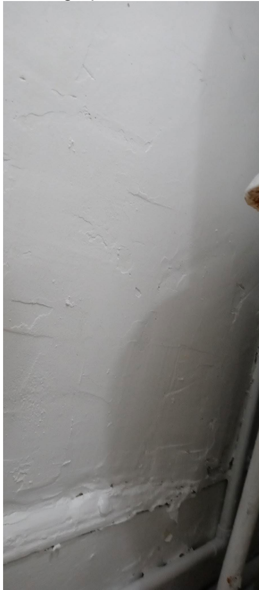
Bathroom Wall B
