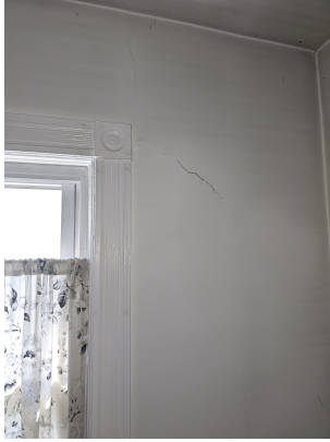
Hazard: Kitchen | Wall | Deteriorated Paint
