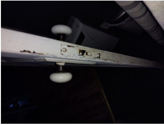
Hazard: Bathroom 1 | Door | Deteriorated Paint
